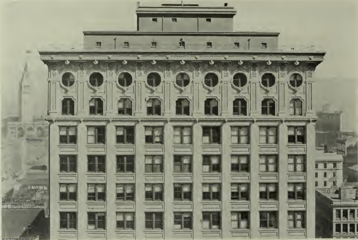
DETAIL OF UPPER STORIES, THE ALASKA COMMERCIAL BUILDING. Meyers & Ward, Architects.
